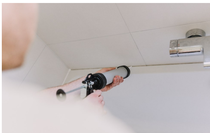
Figure 13. Sealing exterior and interior gaps provides multiple layers of exclusion. Photo: Shutterstock
