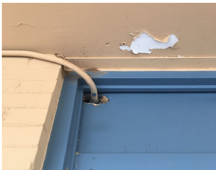
Figure 16. The gap around the wire passing through the door frame needs to be filled. Photo: Shujuan Li, University of Arizona
