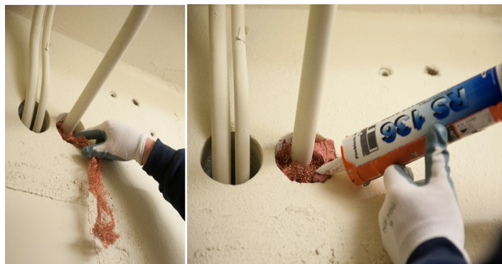
Figure 14. Seal around conduits penetrating walls. Fill gaps with rodent-proof mesh material, then seal with a siliconized acrylic latex or polyurethane sealant. Photo: Lynn Ketchum, Oregon State University
