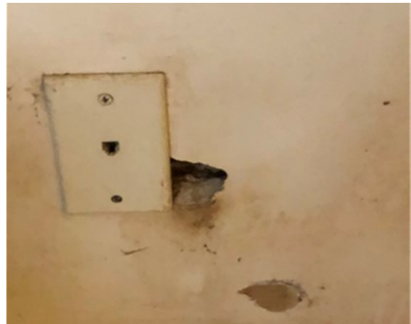
Figure 9. Rub marks can tell us where mice travel. They entered this apartment through this hole from the wall void. Photo: Susannah Reese, StopPests
