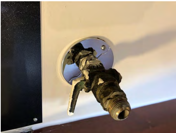
Figure 17. Deny access to wall voids by ensuring collars and escutcheon plates fit around pipes and conduits. This shows a perfectly installed escutcheon plate around a gas line installed during unit turnover. Photo: Susannah Reese, StopPests
