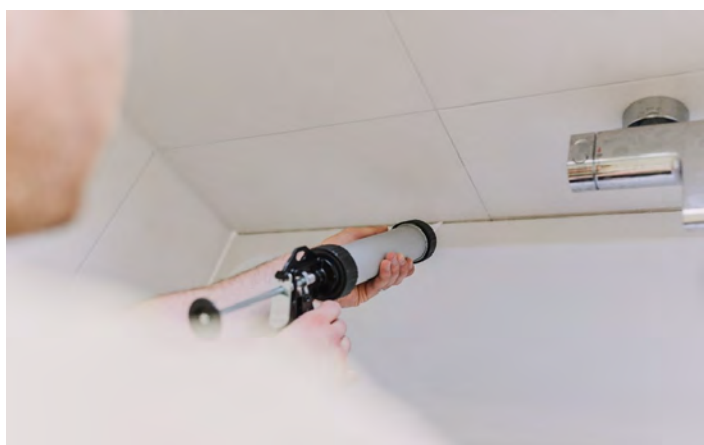
Figure 13. Sealing exterior and interior gaps provides multiple layers of exclusion. Photo: Shutterstock
