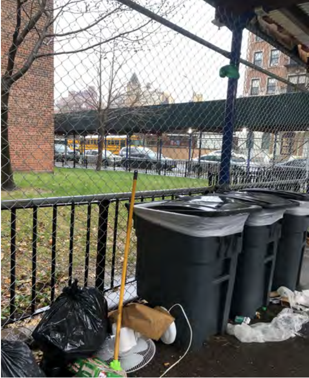
Figure 20. These three trash cans do not have enough capacity for this building and garbage containing food scraps will attract rodents close to the building. Photo: Susannah Reese, StopPests
