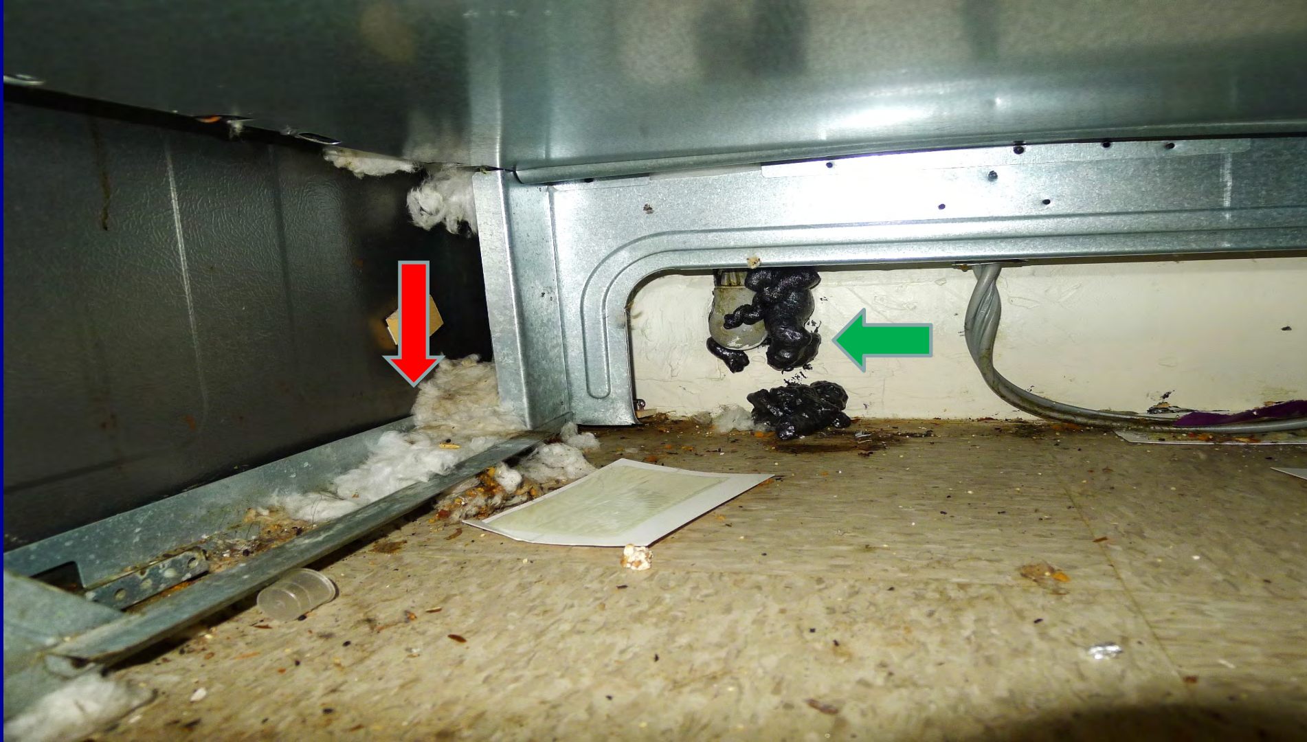
Figure 16. A closer look at Figure 14. Mice living in stoves will drag the batting from the walls and use it for bedding in any nook and cranny of the stove's base –often in the back of the broiler pan's or the bottom pot/pan drawer of stoves. (Red arrow points to a mouse bed. The green arrow points to a amateurish attempt at using cheap foam spray to plug the walls holes that contain the electrical sockets and plugs. Mice actually love the foam for insulations and to make foam beds and the like.
