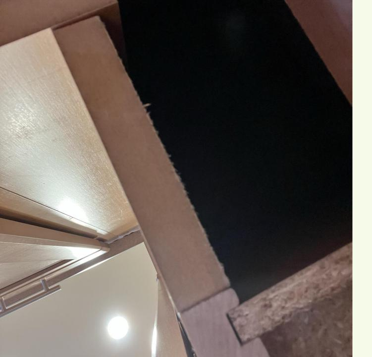
Cabinet designs and installs must avoid open voids like this one, shown from underneath the cabinet above the backsplash, that allow pest access to the space behind the cabinet..
