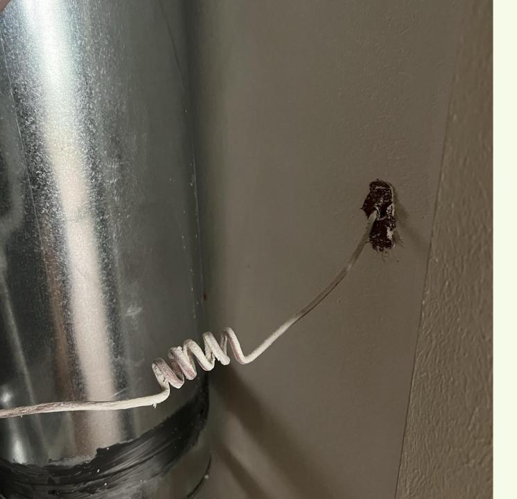
High-risk wiring. Avoid running unprotected wiring across open spaces to reduce damage/need to replace or repair after wiring is snagged and pulled inadvertently.
