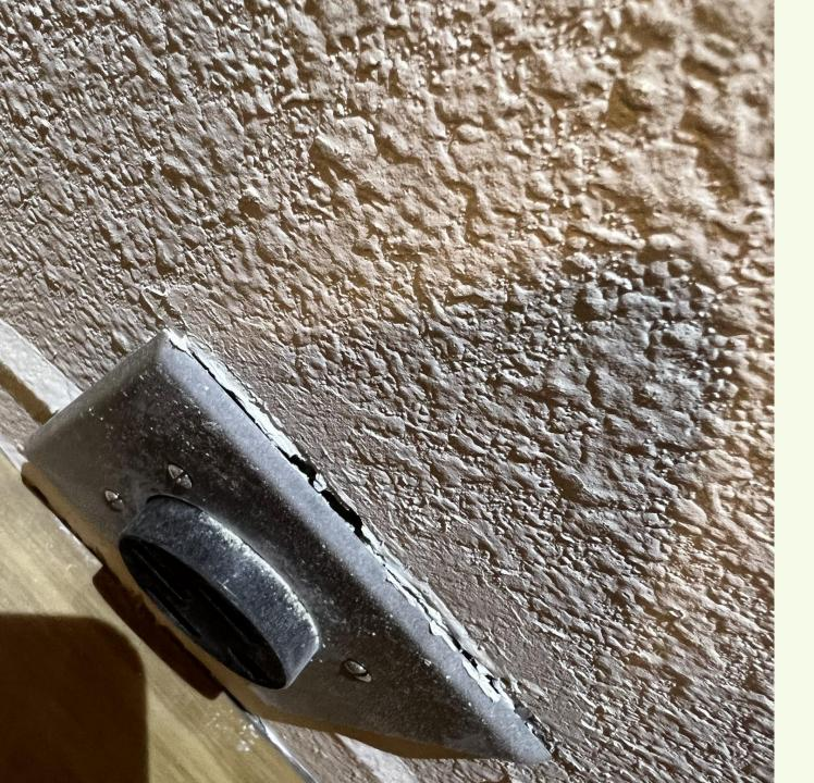
All electrical switch and outlet cover plates need to be tight to the wall, unlike this and many other outlet covers behind appliances, in cabinets.
