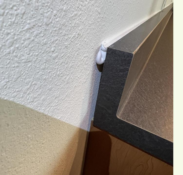
Backsplashes must be completely sealed on tops, sides and exposed bottom portions — not just the junctions that are visible.
