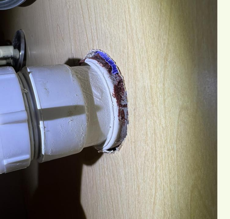
Avoid placing pipe joints where escutcheon plates need to be installed. This joint prevents a standard plate from fitting properly.
