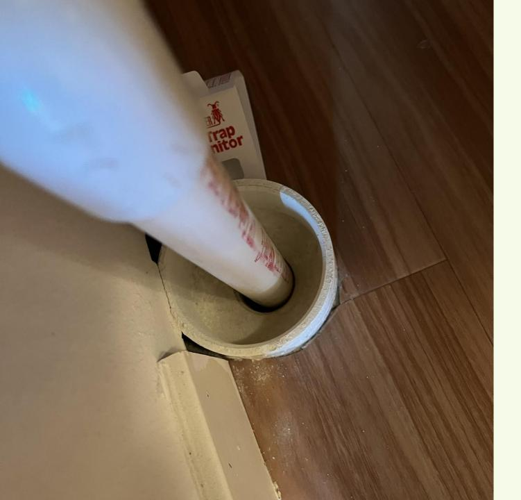
Gaps such as that between the receiving pipe and the entering pipe need to be sealed. If air and liquids must be allowed to pass, stainless mesh can be used to close the gap.
