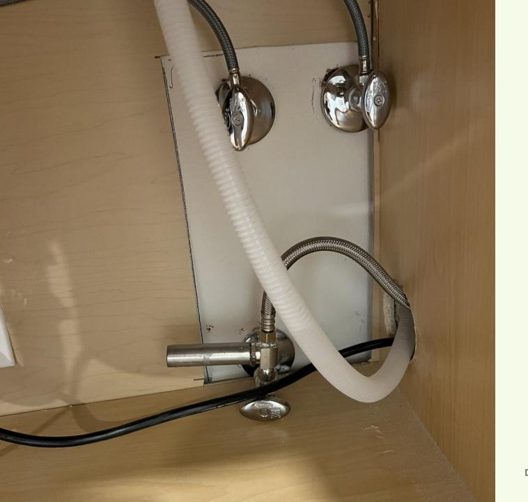
This cabinet has been improperly cut to speed installation.
