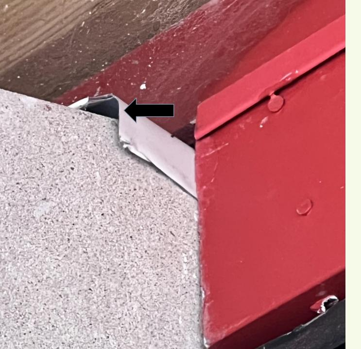
Large gaps in flashing should be stuffed with Xcluder or similar water-permeable material to eliminate pest access/harborage.
