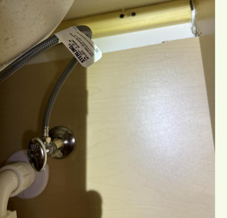
Improper cuts at the top of cabinets, both back and sides, leave wide open access to the void behind the cabinet, and access to the other cabinets, drawers, etc.
