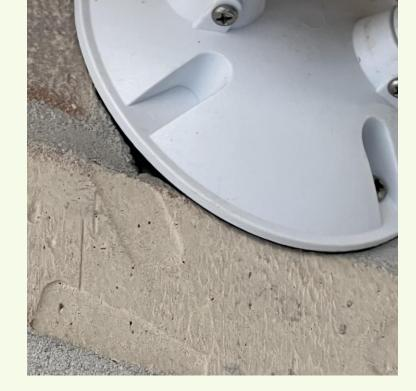
Gaps around all penetrations need to be sealed. There is also an unsealed gap along the top of this siding board.
