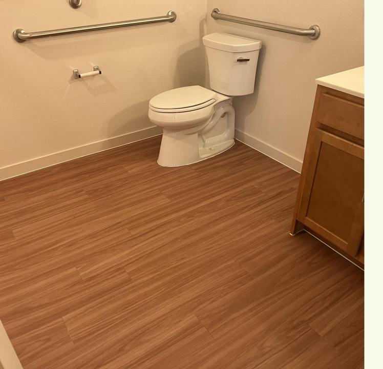
Gaps under baseboards, under toilets and where cabinet bases, kickplates meet floors are all being sealed post-construction to keep debris, spills, urine from penetrating and causing swelling and cracking of particle board, urine odors and other avoidable problems going forward.
