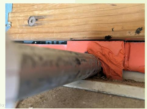
Additional gaps in sealant beads. Picture above right shows fungal growth exposed when the squirrel nest was removed.
