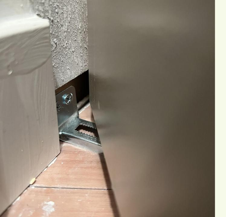
Spaces behind closet door hinges need to be sealed to eliminate pest access to the wall void and avoid accumulation of debris in the void.
