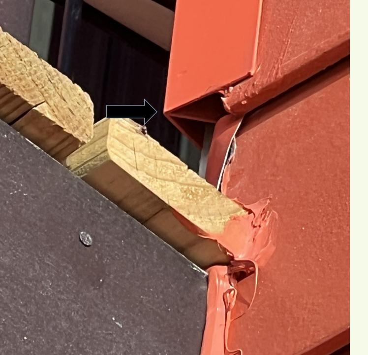
Large gaps at lower (and likely also upper) ends of corner bead need to be stuffed, I use Xcluder mesh secured with silicone sealant. Xcluder allows air and water to escape.
