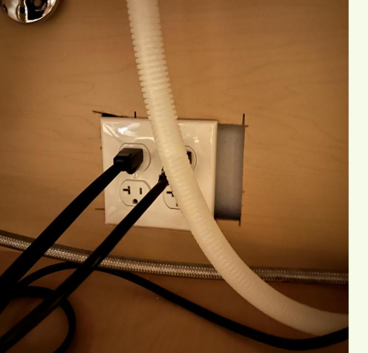
Poorly measured and cut openings must be avoided, and correctly when they occur. This provides pest access and also violates building codes.
