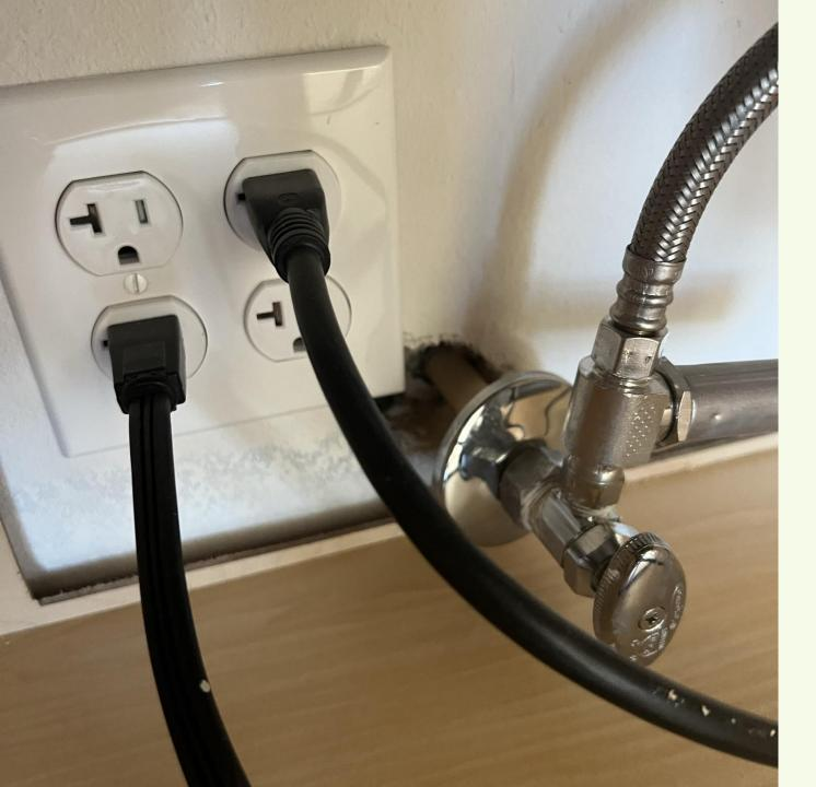
Overlap with electrical boxes/cover plates also need to be avoided to enable proper sealing of escutcheon plates.
