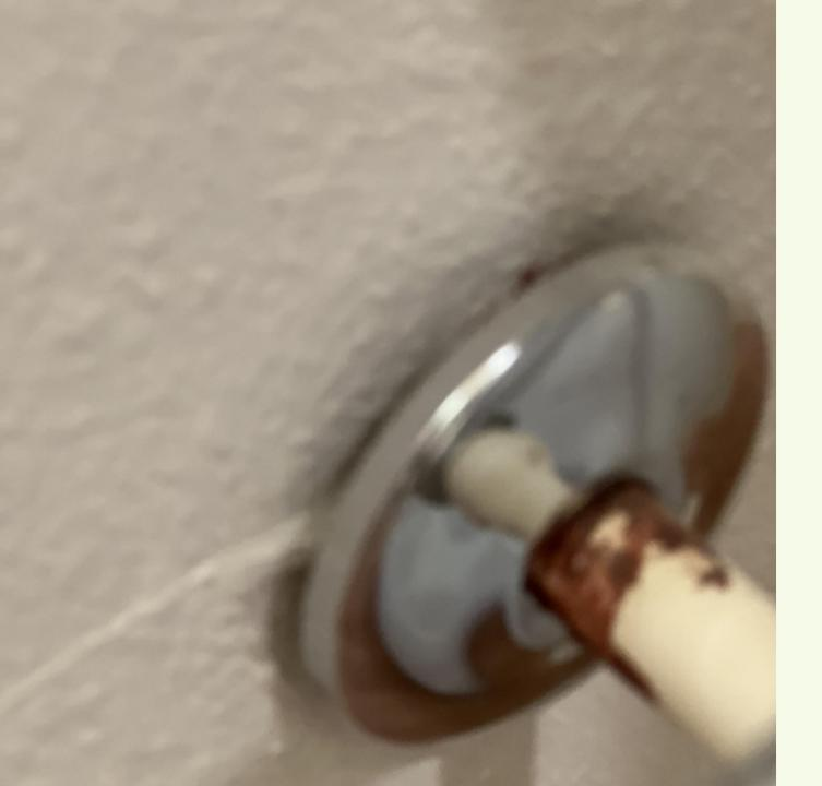
Escutcheon plates need to be firmly sealed to the wall with elastiomeric sealant such as silicone. The pipes they encircle need to be completely free of fire caulk to allow the plate to be moved against the wall to ensure a tight fit.
