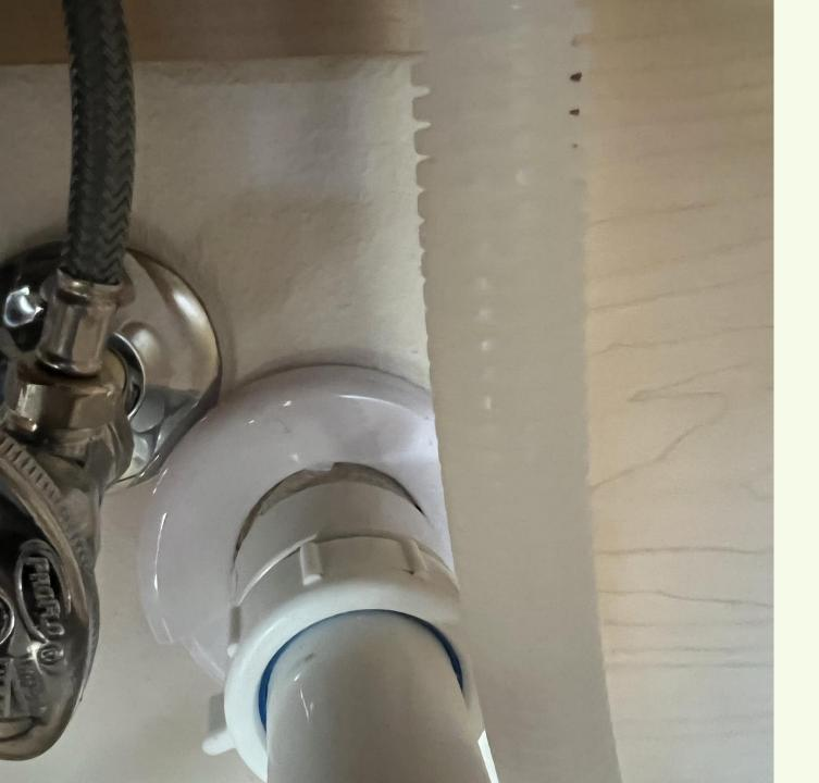
Undersink plumbing penetrations need to be placed so that escutcheon plates can be installed without overlap.
