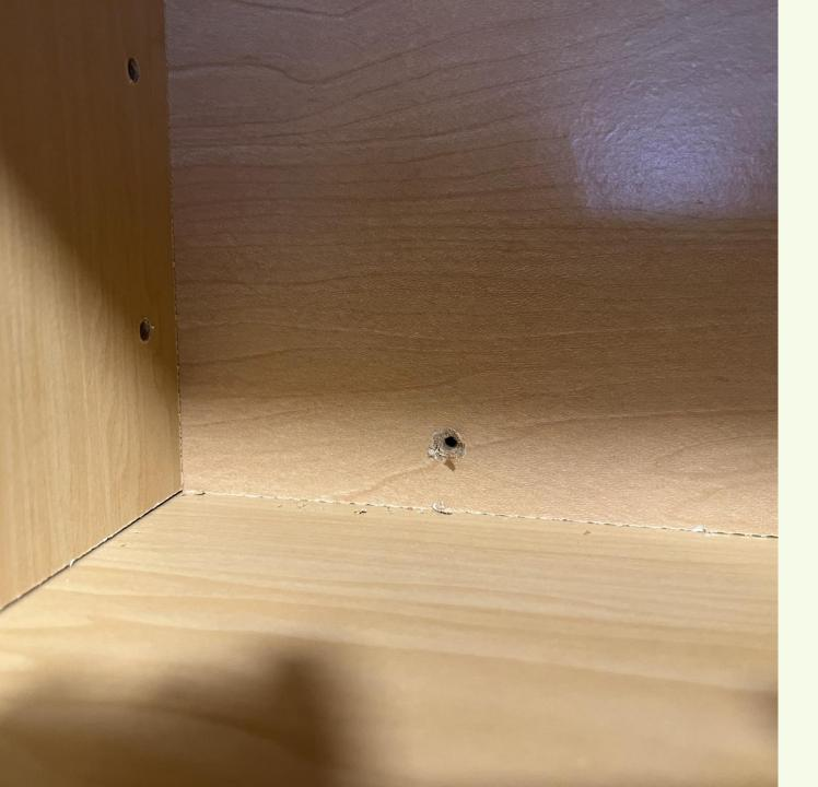
Blind screw holes need to be sealed to prevent pest access.
