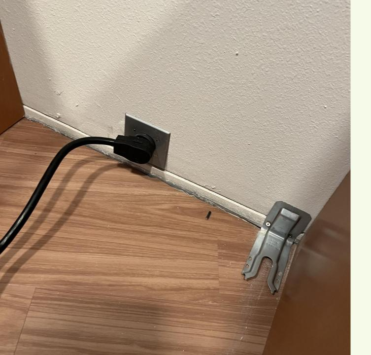
Baseboard areas behind all appliances including stoves, fridges and dishwashers need to be complete with baseboard and elastiomeric sealant where needed to close all gaps where food may accumulate, spills may contact drywall and pests might access wall cavity.
