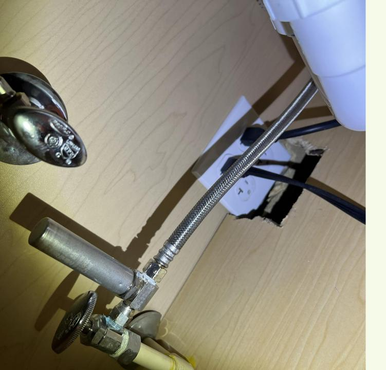
This outlet box was installed improperly and the carpenter cut out the base of the cabinet to accommodate the error rather than have it fixed properly.
