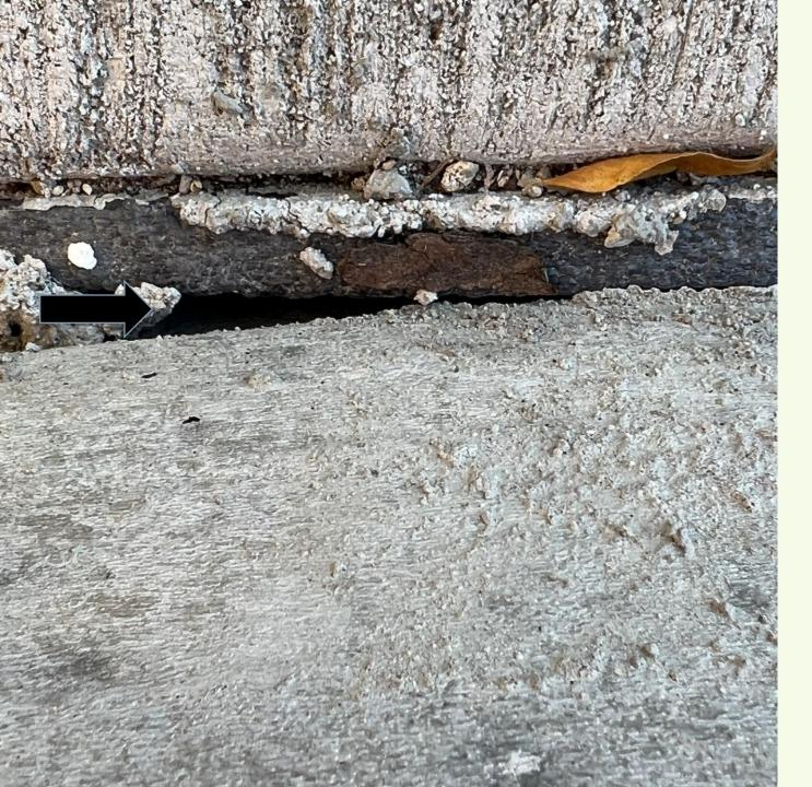
The gap in this expansion joint is likely to lead to water penetration which may be extensive enough to cause concrete to crack when that water freezes. It's also large enough to allow small rodent entry with potential for burrowing.
