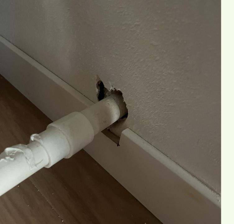
Most penetrations for these HVAC condensation drains were unsealed, proving open access to the wall void.
