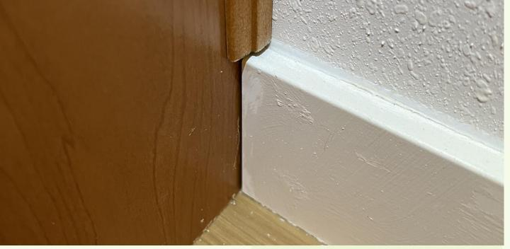
Gaps in baseboards need to be sealed to prevent food, liquids and other debris from accumulating, and prevent pest access to the wall cavity behind the baseboard.
