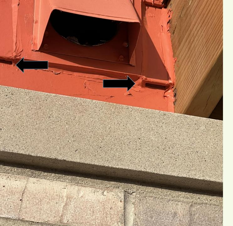
Additional large gaps between siding boards. This gap is large enough for bats or mice to enter. Can they access a cavity once they get behind the siding? We don't know and so have to assume yes and seal these up.
