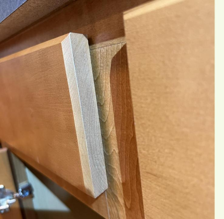
Cabinet designs should avoid unnecessary gaps such as these behind false drawer fronts on under sink cabinets.
