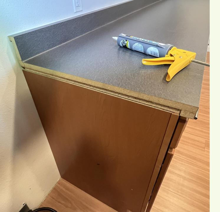
Laminate must be firmly attached to all cut ends of countertops to prevent moisture being absorbed into the particle board and swelling and cracking.
