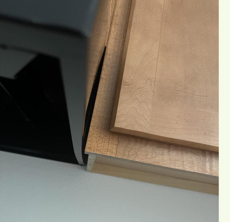
Gaps in upper cabinets that can't be avoided in the design stage should be boxed in top and bottom. Small gaps can be sealed with elastiomeric sealants.
