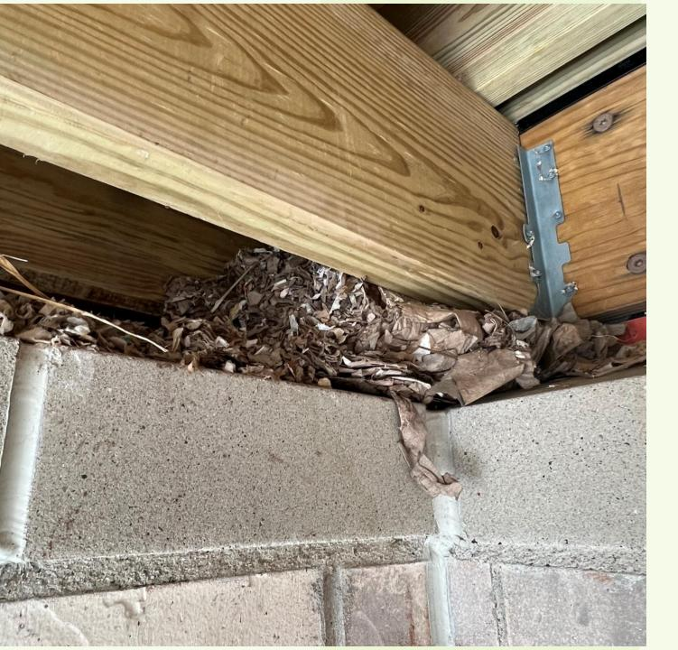
Design elements that create protruding ledges or in this case a protected nook invite bird roosting and nesting, and rodent nesting. These design features should be avoided wherever possible.
