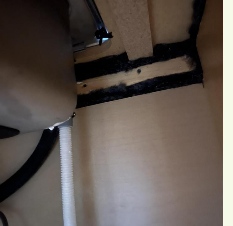
Another shot of sealing with Xcluder secured in place with sealant.
