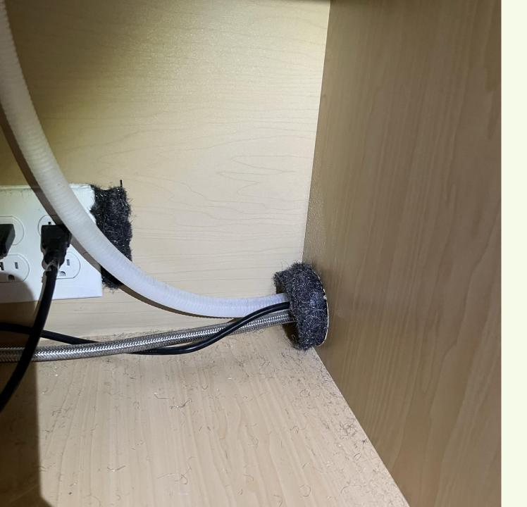
We used DAP silicone sealant and Xcluder stainless steel mesh to seal undersink cabinets post-construction.
