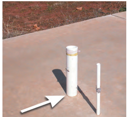
Figure 14. In slab construction, termites often enter the structure via gaps (arrow) that develop between utility pipe penetrations and concrete.
