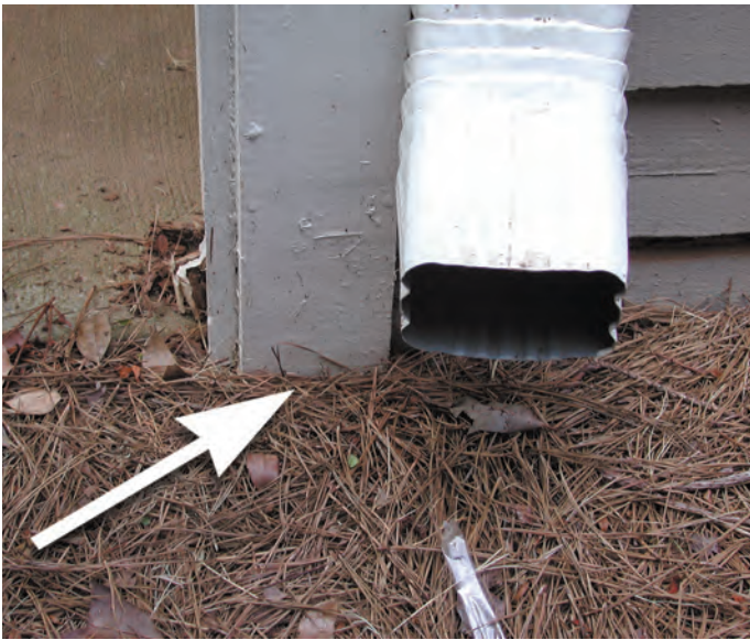
Figure 22. Wood to-ground contact (arrow) is a recipe for termite infestation. In this picture, wood is in contact with the ground in close proximity to where a gutter vents directly into mulch, resulting in persistently moist soil. Note also mulch piled next to the structure's siding
