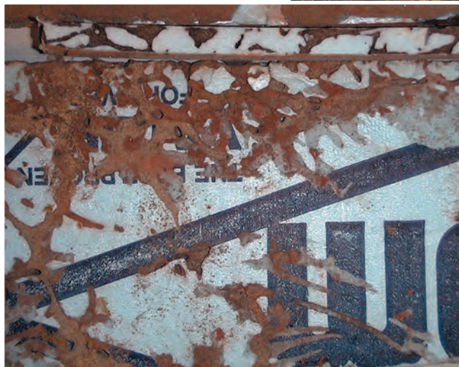
Figure 19. Some construction types, especially EIFS (top), make structures more vulnerable to infestation because they allow termites an undetectable access route into the structure by tunneling through the insulation itself (bottom).
