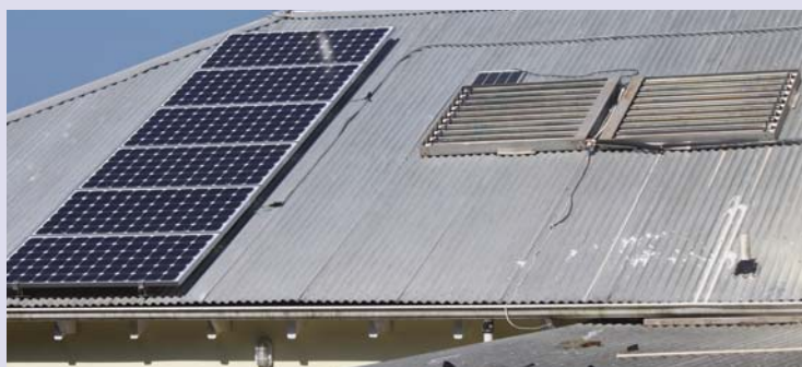
Solar Water Heater and Photovoltaic (Water and Electricity) Collectors
