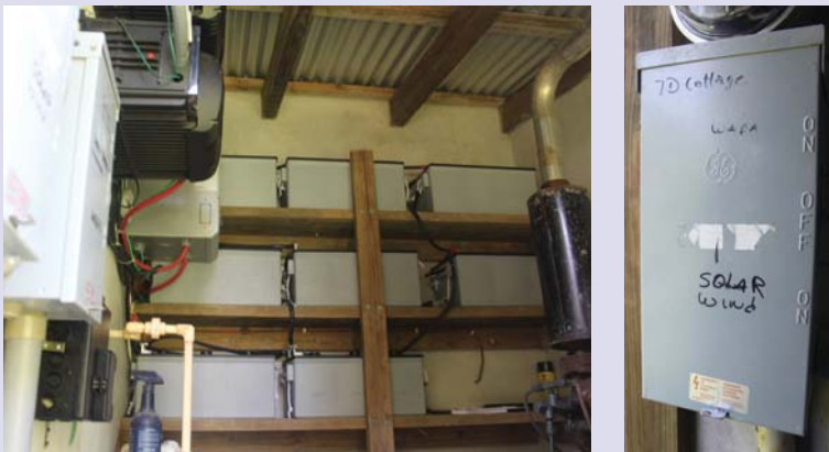
Photovoltaic Storage Batteries and Switch
